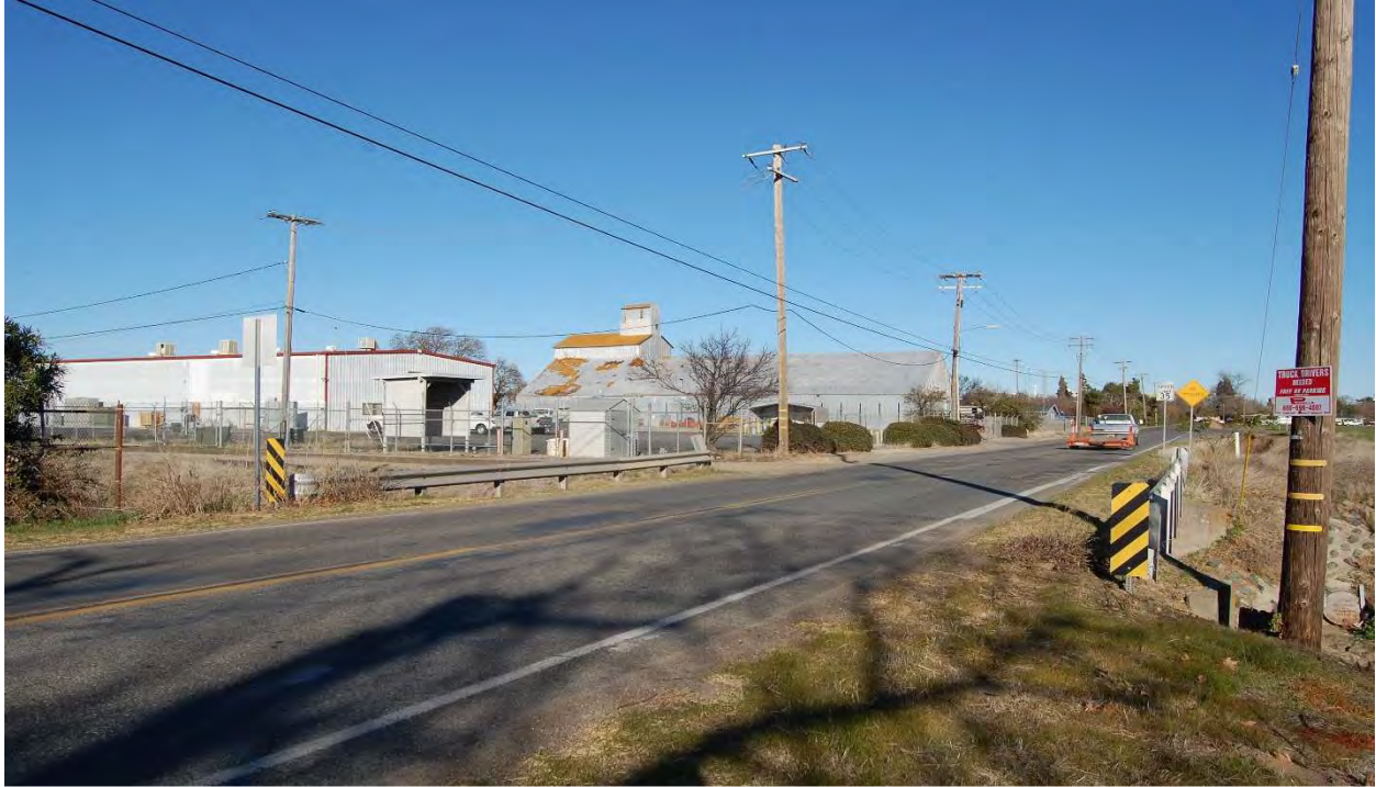
PHOTO 3: BRIDGE CROSSING OVER MAIN DRAINAGE CANAL AT WEST BIGGS GRIDLEY ROAD, LOOKING NORTH
