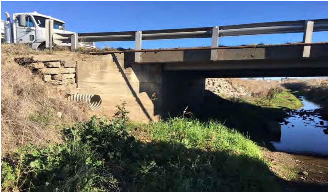
PHOTO 4: MAIN DRAINAGE CANAL AND BRIDGE ABUTMENTS, LOOKING EAST
